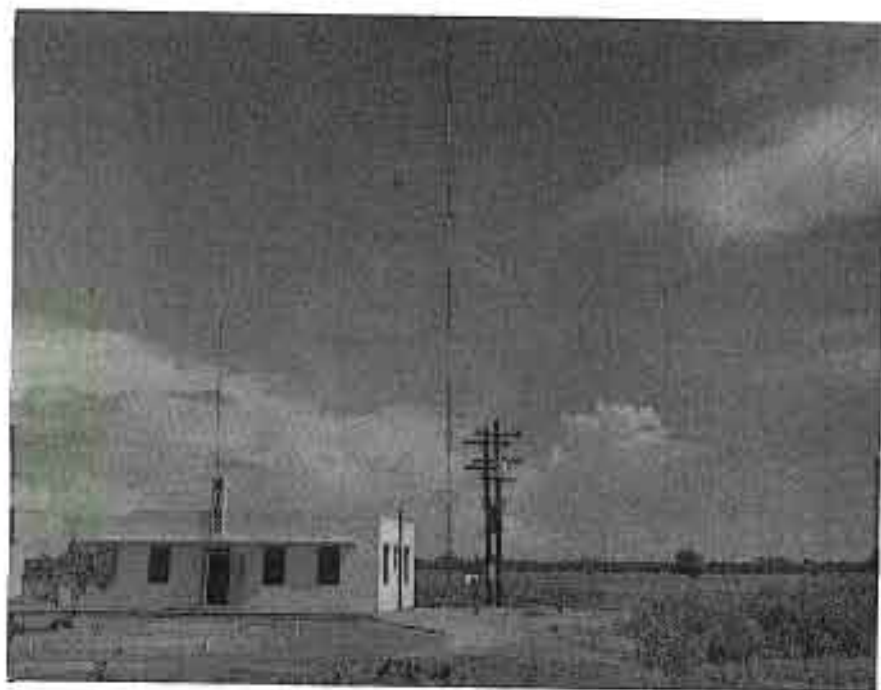
Above, view of WBS building in San Juan, Puerto Rico, which houses 10 kw a-m transmitter, operating on 740 kc. The building is located seven air miles from downtown San Juan. A two-tower directional antenna array is used to provide a cardioid pattern; full 10-kw power is used for day and night service. Below, Carlos Rafael Mercado, WBS engineer, inserting a rectifier tube in the main rectifier power supply of the transmitter.
